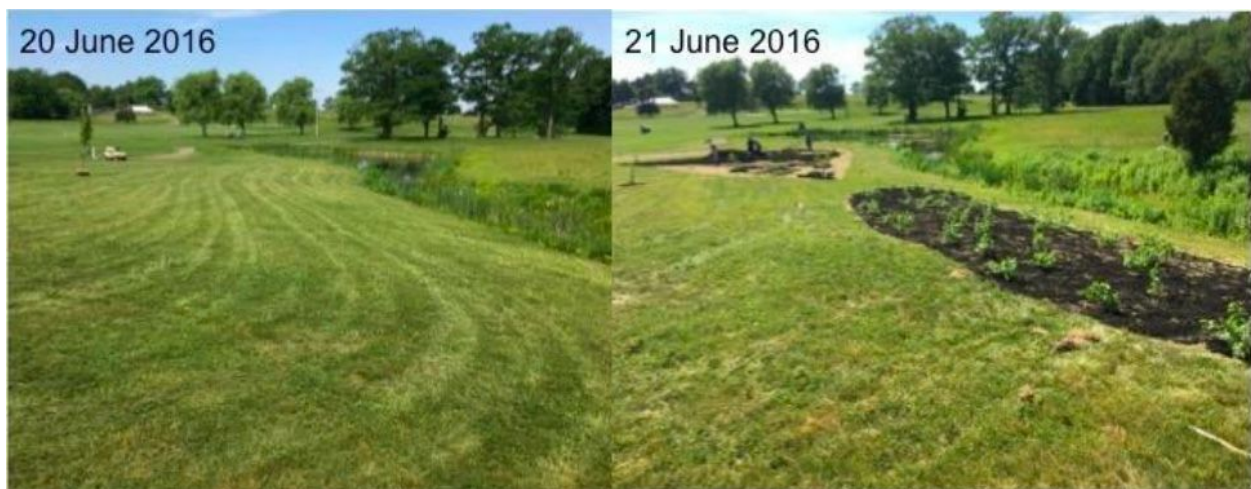
Pre- and post-restoration photos of a riparian buffer area in North Hampton, New Hampshire. Photos provided by New Hampshire Sea Grant.
